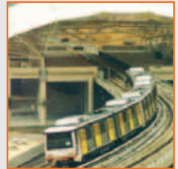
INTEGRATED SCADA MALAYSIA
