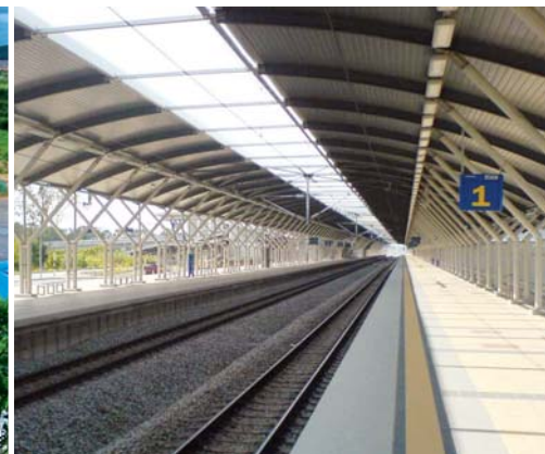
Railway Utilities Monitoring
